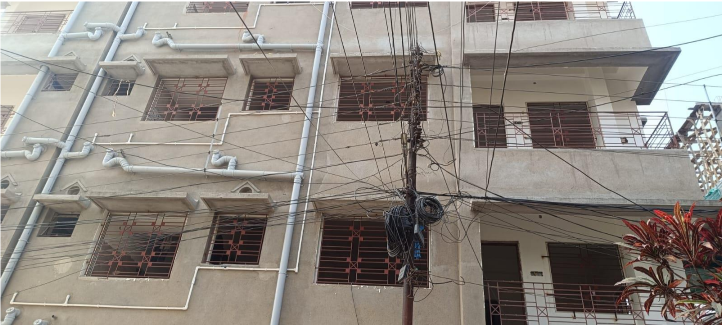
External Construction/Infrastructure Photo
